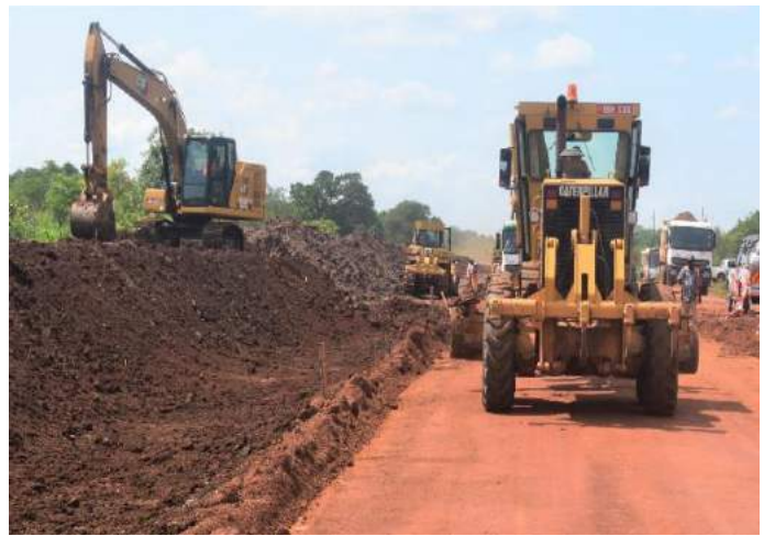
Atiak – Laropi road is being upgraded from gravel to bitumen standard.
