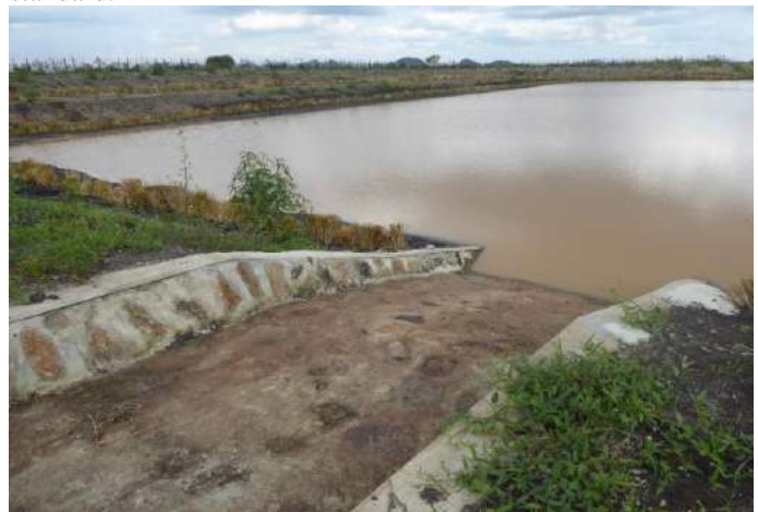
Water source protection measures at the valley tanks.
