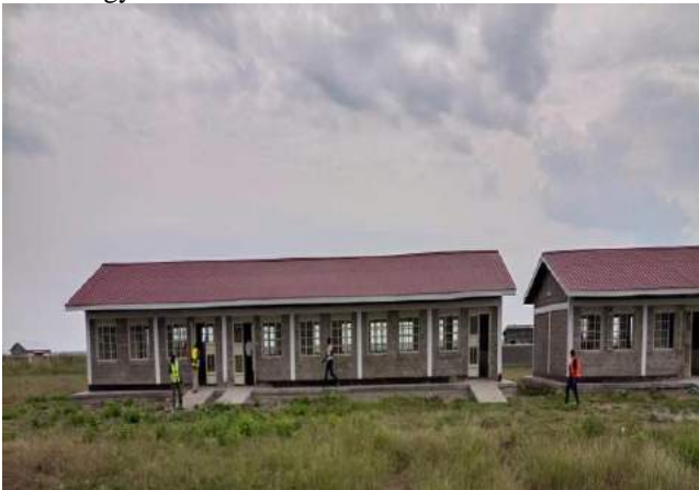
Classroom blocks constructed at Bunambutya settlement for disaster victims from Elgon sub-region
