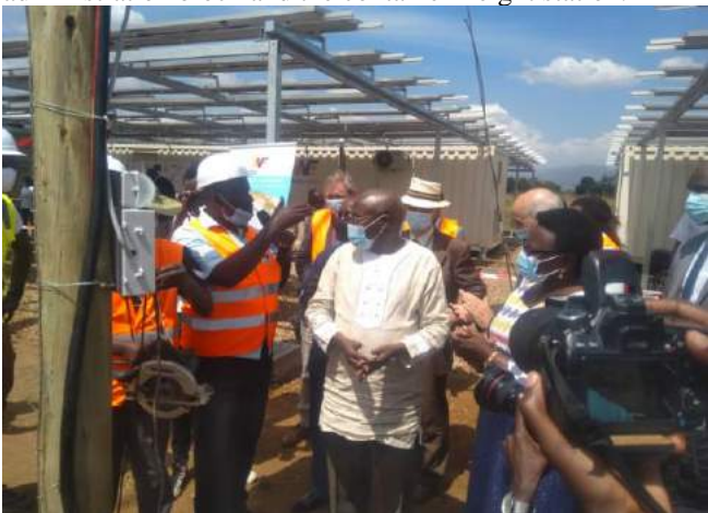
Solar PV Generation and storage systems in Lamwo under mini grids construction
