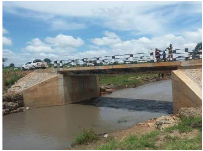
Kopu bridge in Koboko District constructed under the project
